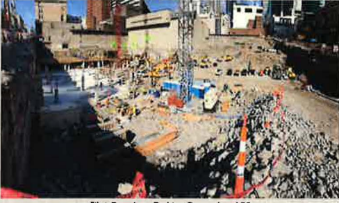
5 th + Broadway Parking Garage Level B2
